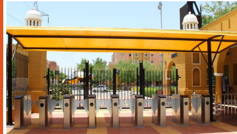
RFID smart access control at Entry/Exit (Flap Barriers)
